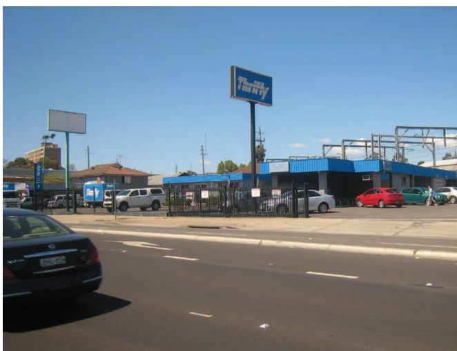
View from site south across Parramatta Road
