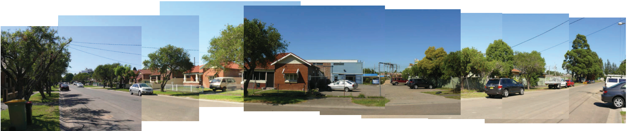
Panoramic view of site from Victoria Street (north of site)
